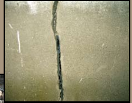
Foundation Cracks
