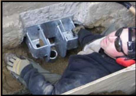
Foundation Underpinning
